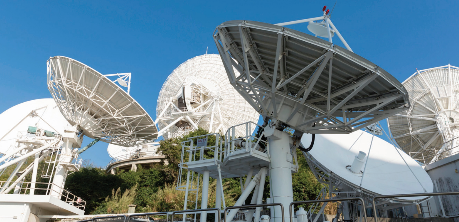
Oxford Falls Teleport, Sydney, Australia. Photo courtesy Telstra ●●●
